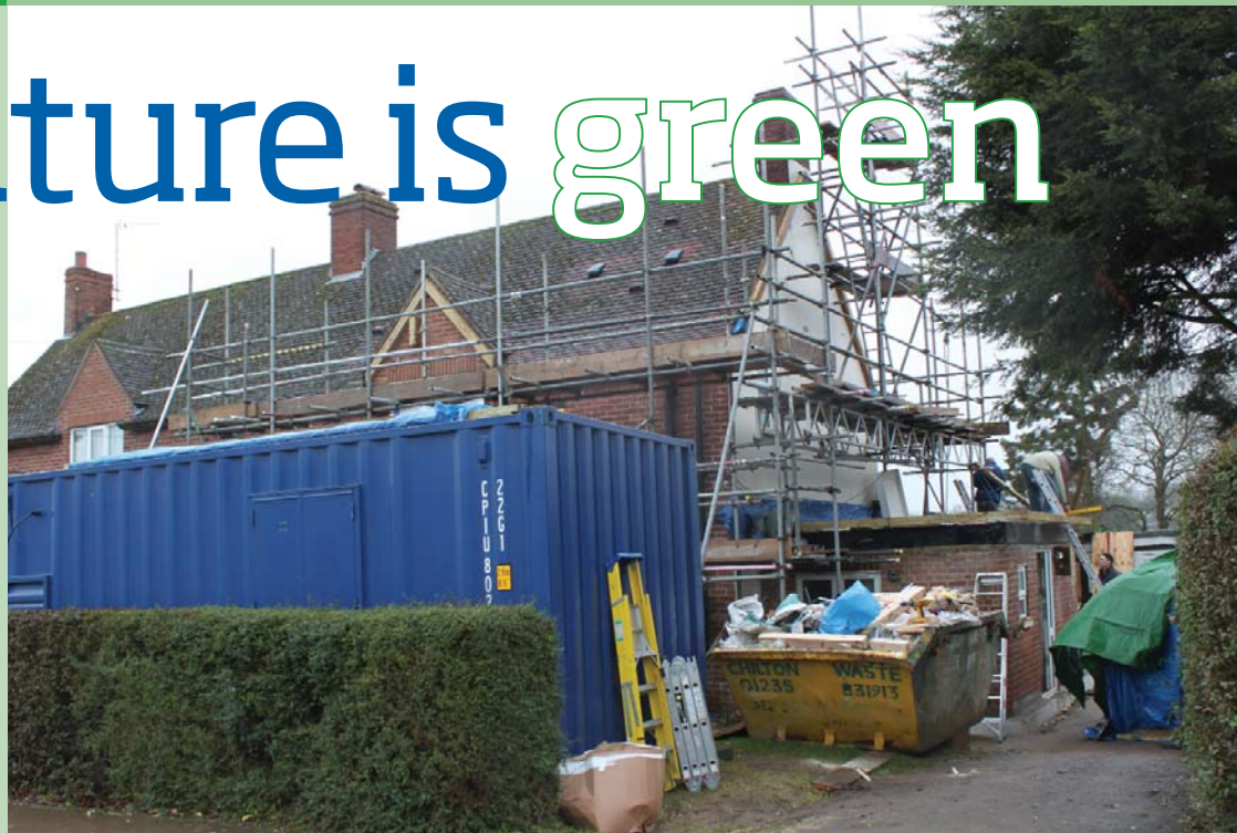
Work starts on the retrofit at Manor Crescent in Compton, Berkshire.
