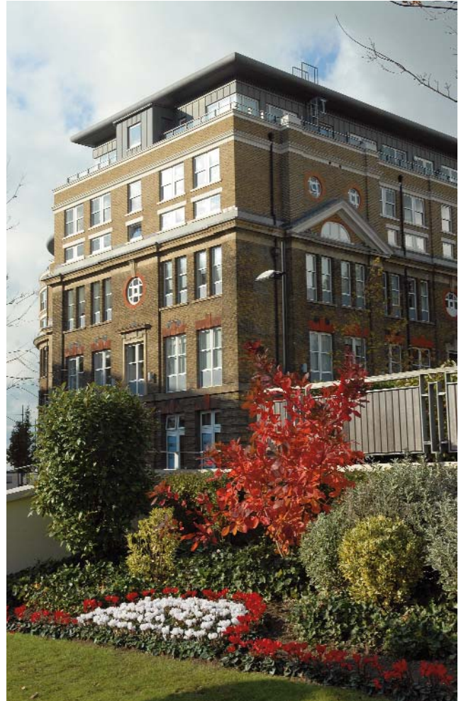
Base 18 at our Royal Arsenal scheme in Woolwich.
