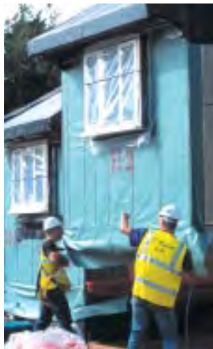
Installation of one of the modules at Kettle Drive near Folkestone.
