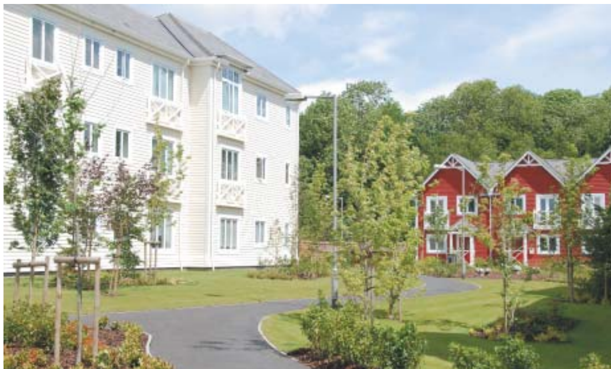
The first 40 homes of our development at Holborough Valley, Snodland, Kent were completed this year. Of the 1,000 eventual homes, 25 per cent will be affordable.
